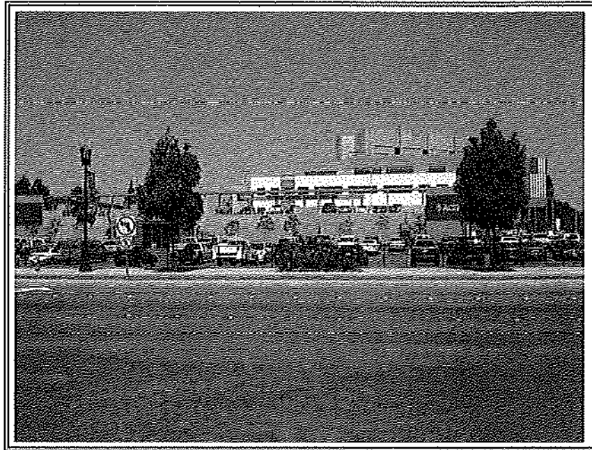
Looking easterly toward the subject from N. Magnolia Avenue.
