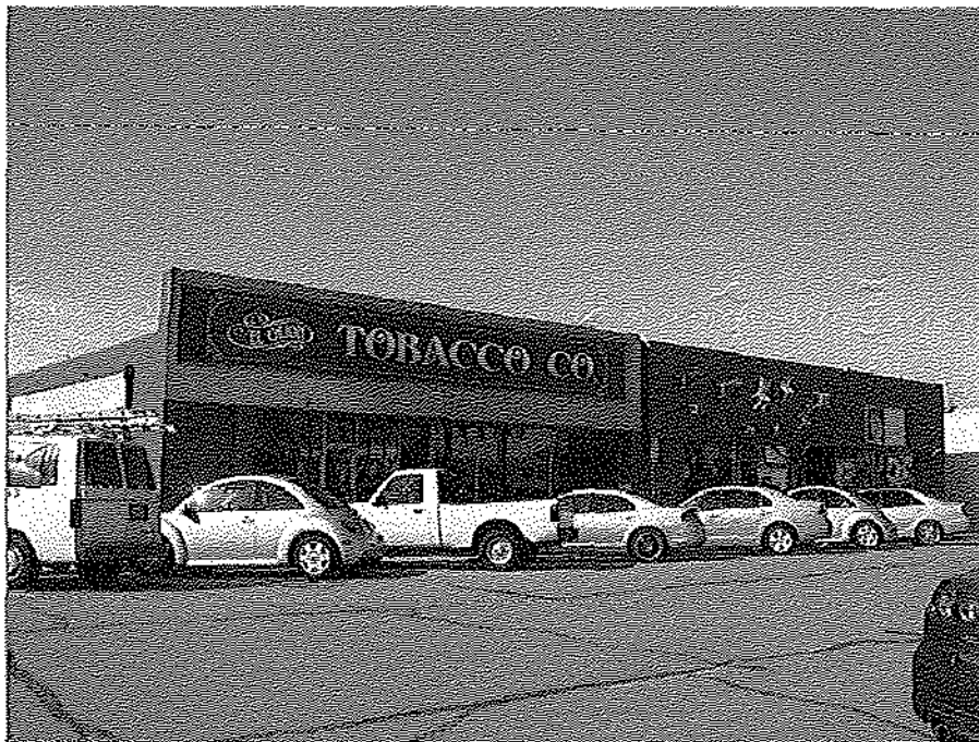
Looking southwesterly toward site from Rea Ave.
