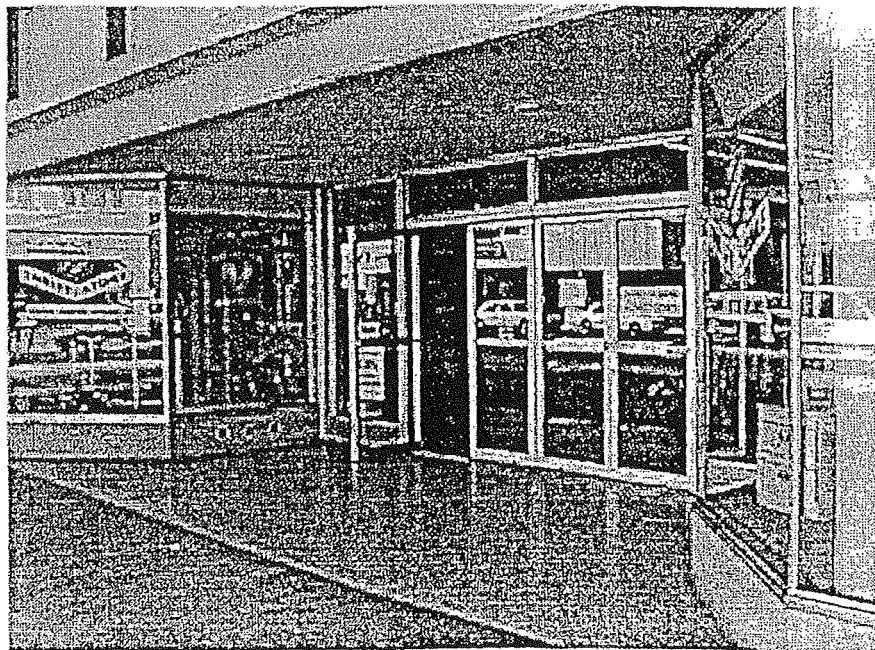
Extruded aluminum window sash and doorjamb epitomize this buildings era, circa 1955.
