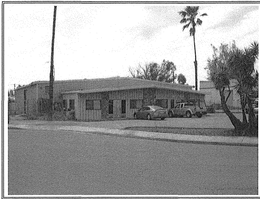
Looking easterly toward the front of 549-555 Raleigh Avenue.
