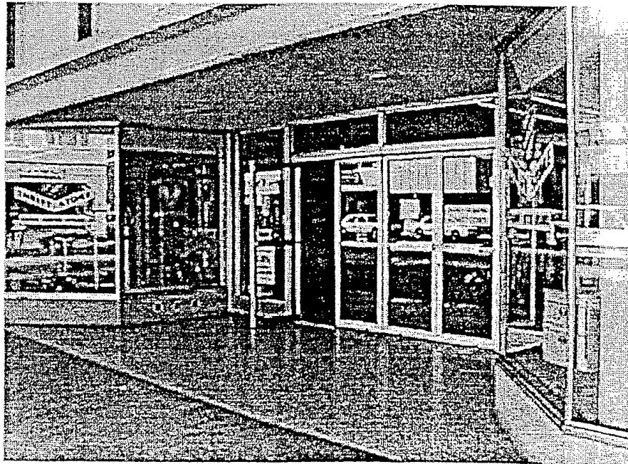
Extruded aluminum window sash and doorjambs epitomize this buildings era, circa 1955.
