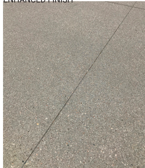
STANDARD GRAY CONCRETE WALK WITH ENHANCED FINISH
