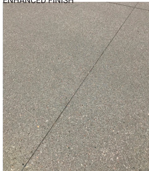
STANDARD GRAY CONCRETE WALK WITH ENHANCED FINISH
