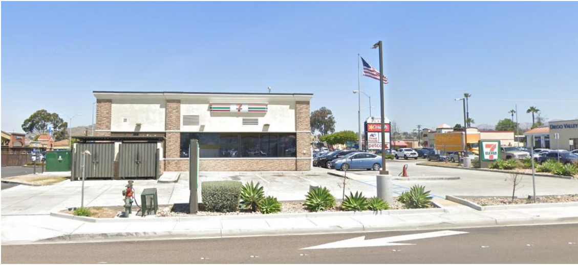
3. 500 N. 2nd Street: view looking north at the south side of the subject property.
