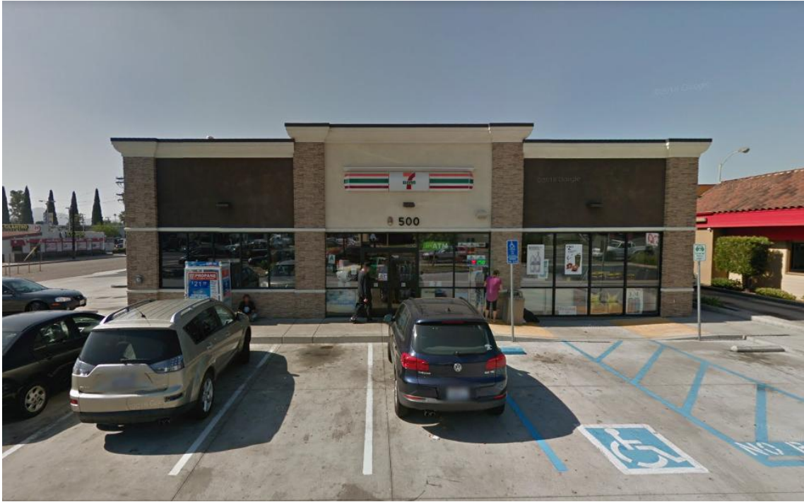
1. 500 N. 2nd Street: view looking west at the front entrance of the subject property.
