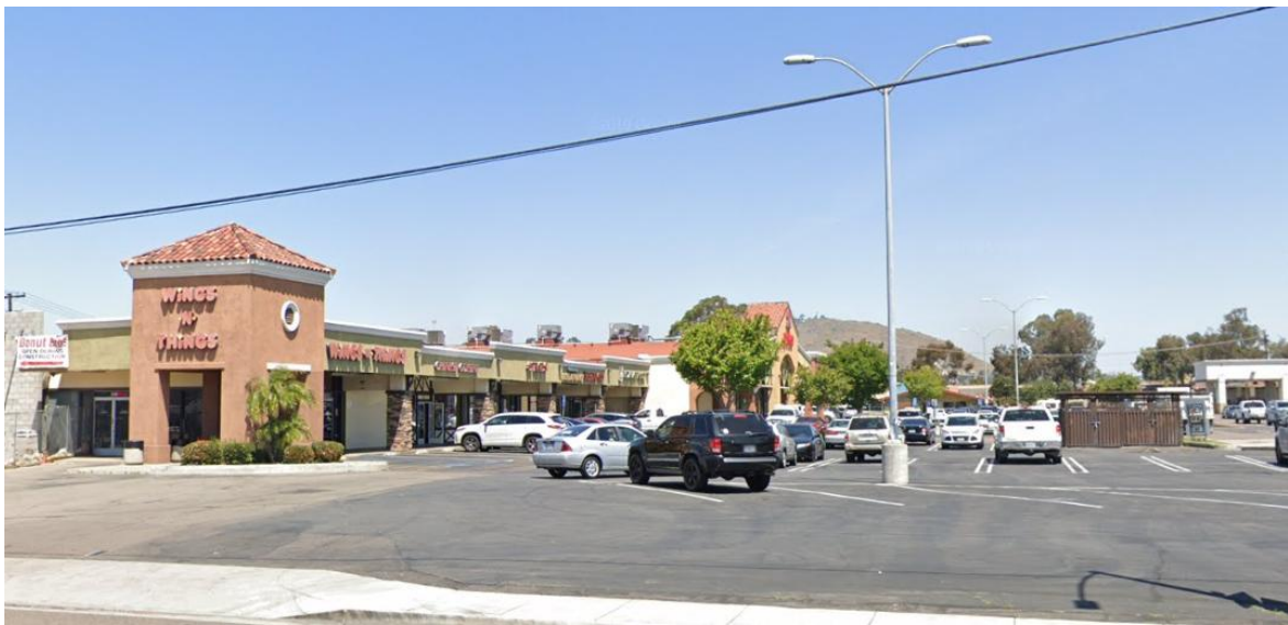
13. 500 N. 2nd Street: view looking northwest at the neighbors to the west of the subject property.
