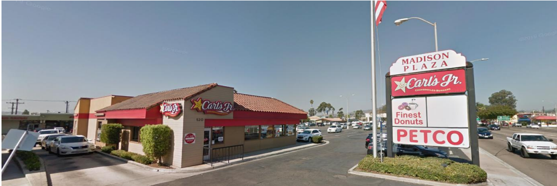
16. 500 N. 2nd Street: view looking north at the neighbors to the north of the subject property.
