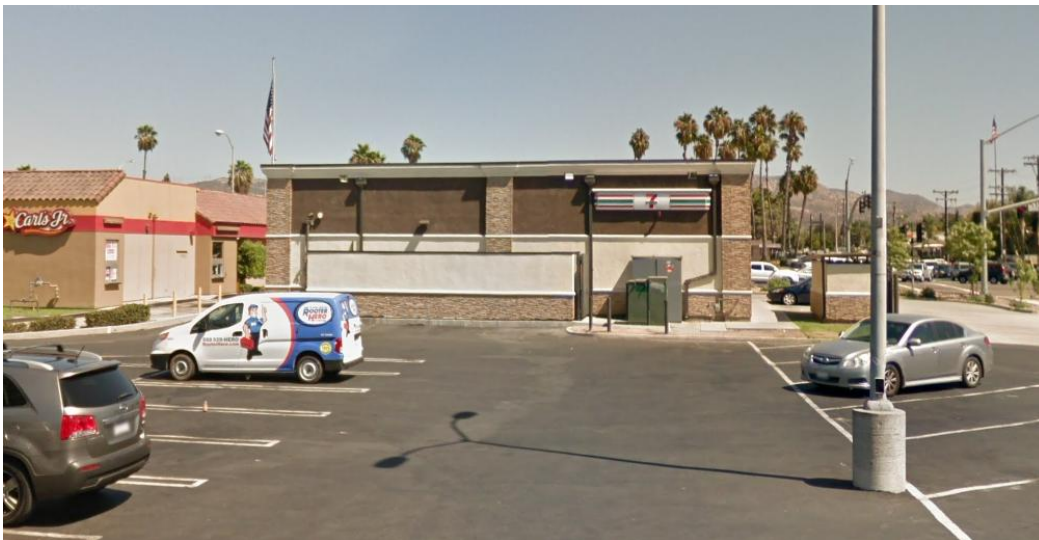
5. 500 N. 2nd Street: view looking east at the west side and rear of the subject property.
