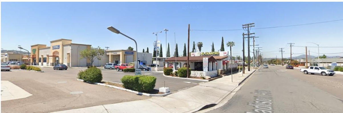
18. 500 N. 2nd Street: view looking southwest at the neighbors to the west of the subject property.
