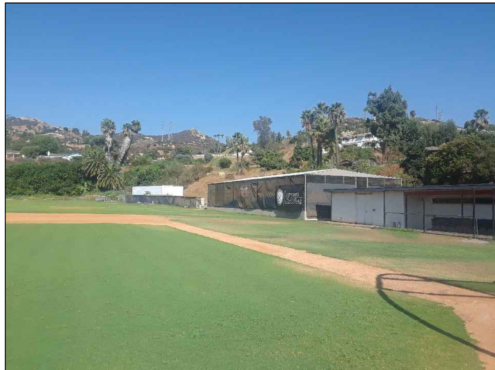
EXISTING BATTING CAGE AND DUGOUT *NO CHANGES TO DUGOUTS OR BATTING CAGE
