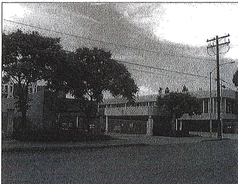
Looking northwesterly to site. Lexington Sr. Apts to left.
