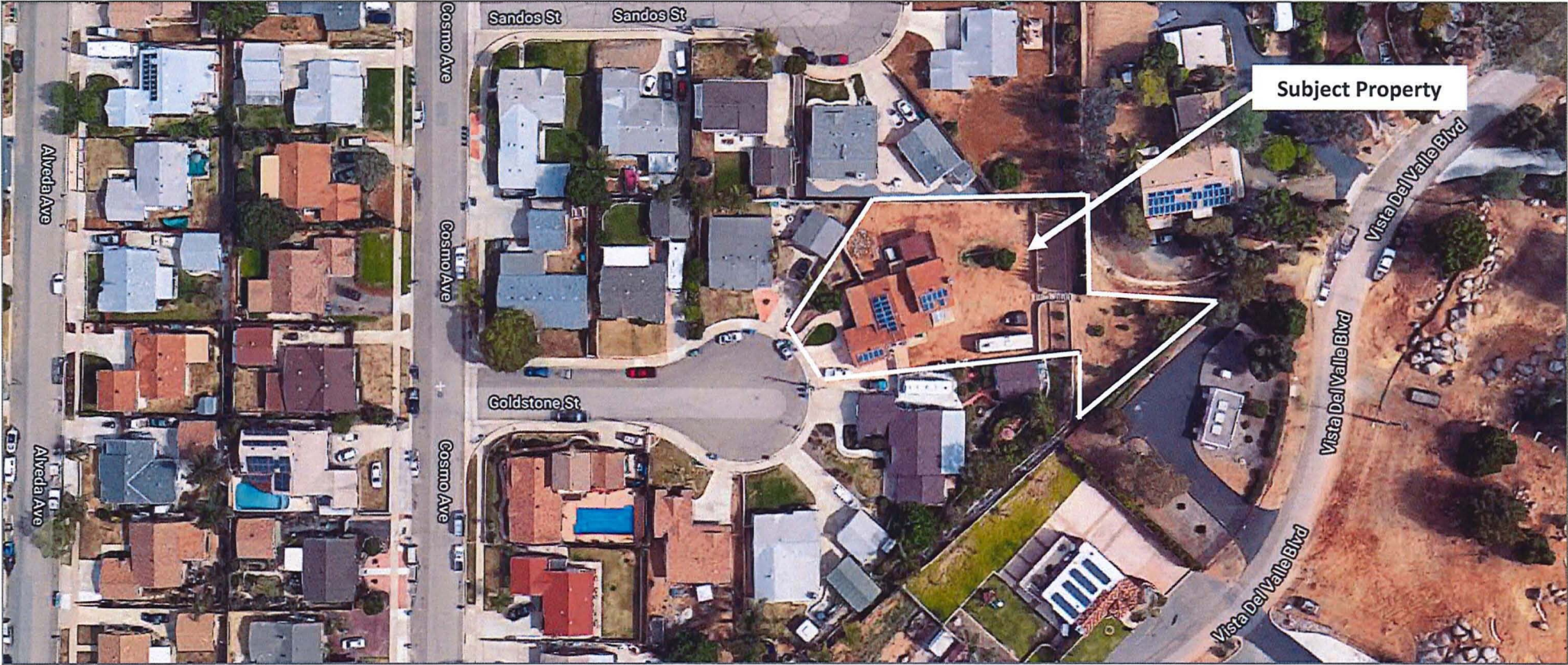
Aerial Image – 1680 Goldstone Street
