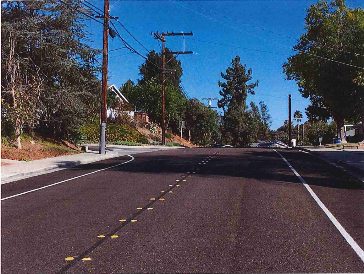
Northbound on Brockton Street south of Katherine Street
