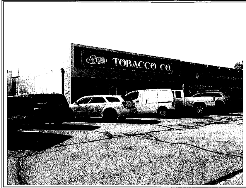
Looking in a southwesterly direction toward the front and eastern side of the subject from Rea Avenue.
