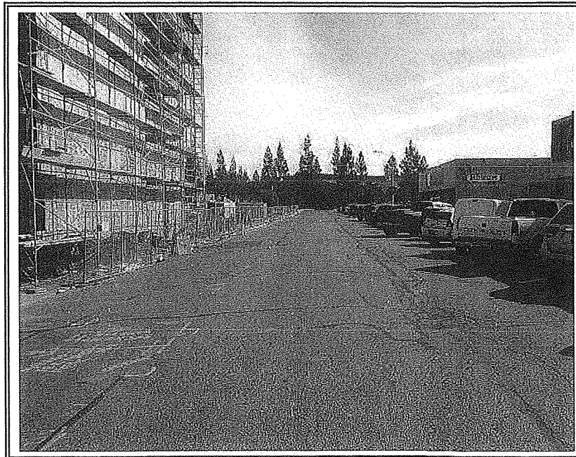
Looking in an easterly direction along Rea Avenue. The subject is located on the right side of the photograph
